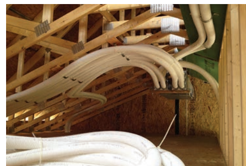
Top left: The first floor features an open layout. The kitchen and dining area is set up for maximum efficiency for meal preparation and clean-up. Top right: The view of the Holyoke Range from one of the second story windows. Above: The heat/energy recovery ventilation system.
