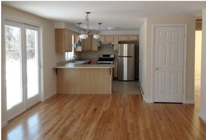
Integrity installed the hardwood floors in this modular home. The kitchen features standard cabinets and countertops.
